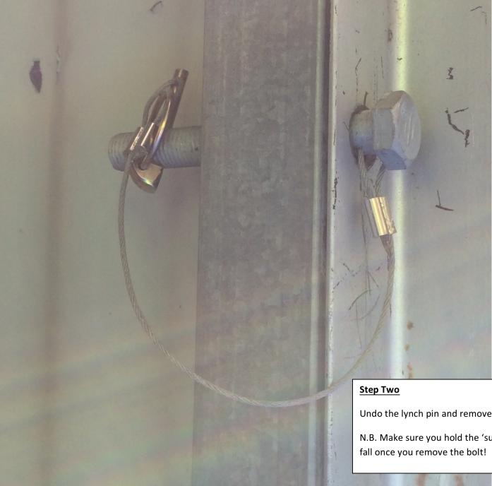
Undo the lynch pin and remove the securing bolt.
